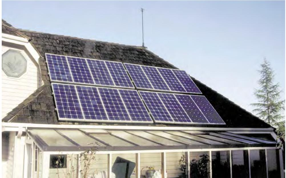
Sixteen AstroPower PV modules, for a total of 1,920 rated watts, are mounted on the south-facing roof above the greenhouse.
